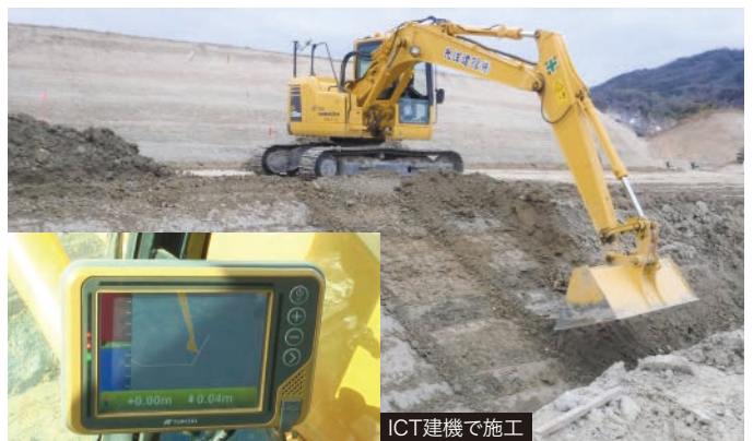
ICT建機で施工
